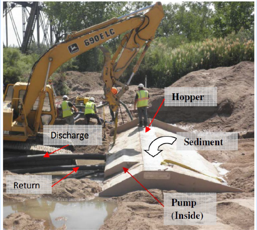
Components of the Sediment Collector™ at the Fountain Creek, CO install (Tucker et al., 2015) MSAC utilized information from the Omaha District's RSM program proposal for portions of this report.
